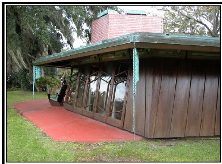
Auldbrass bedroom - note the angle of the walls and doors (which must be opened outward), and the beautifully stylized “Spanish Moss” copper downspouts
