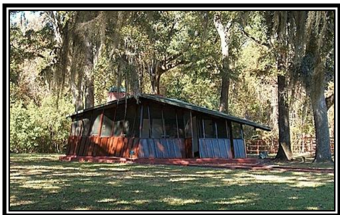
Auldbrass Plantation Guest House - note the 81° angle of the walls, rather than the standard 90°
